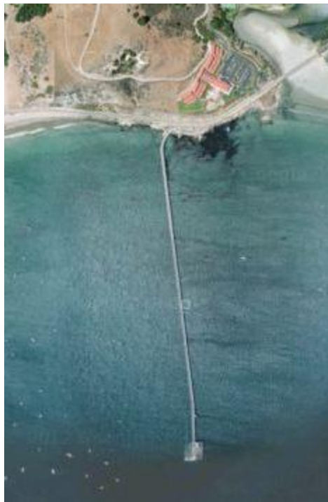
Figure 5.2: Cal Poly Pier, Avila Beach, CA.
